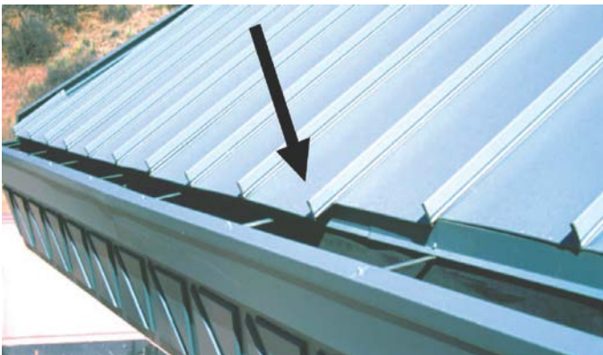
▲ Most two-piece clip designs provide for differential movement within the clip itself. The base is fixed to the structure and the top flange into the panel seam. The top does not move relative to the seam, preserving the integrity of seam sealants.
