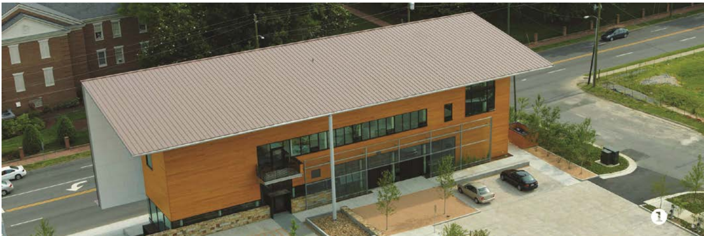
▲ VMZ Double Lock Standing Seam Panels in Pigmento Red from VMZINC were used on the AIA North Carolina chapter building in Raleigh.
