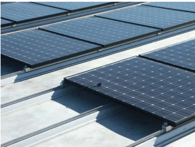
▲ Metal roofing can make use of special seam-clamping hardware that grips the standing seam without puncturing the membrane. Seam clamps have made metal roofing a preferred roof type for mounting photovoltaic solar arrays.
