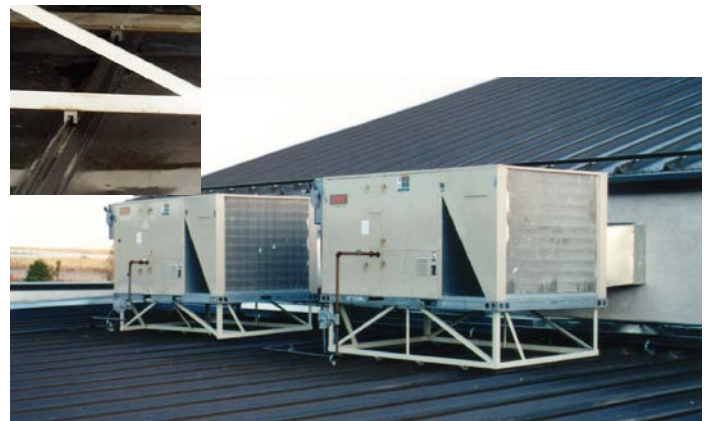
▲ A frame-mounted HVAC unit can be supported without roof penetration by using seam clamps.
