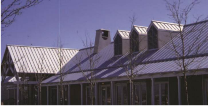
▲Cosmetic surface stains that detract from the appearance of unpainted Galvalume in steep applications can be minimized by using Acrylume or Galvalume Plus.
